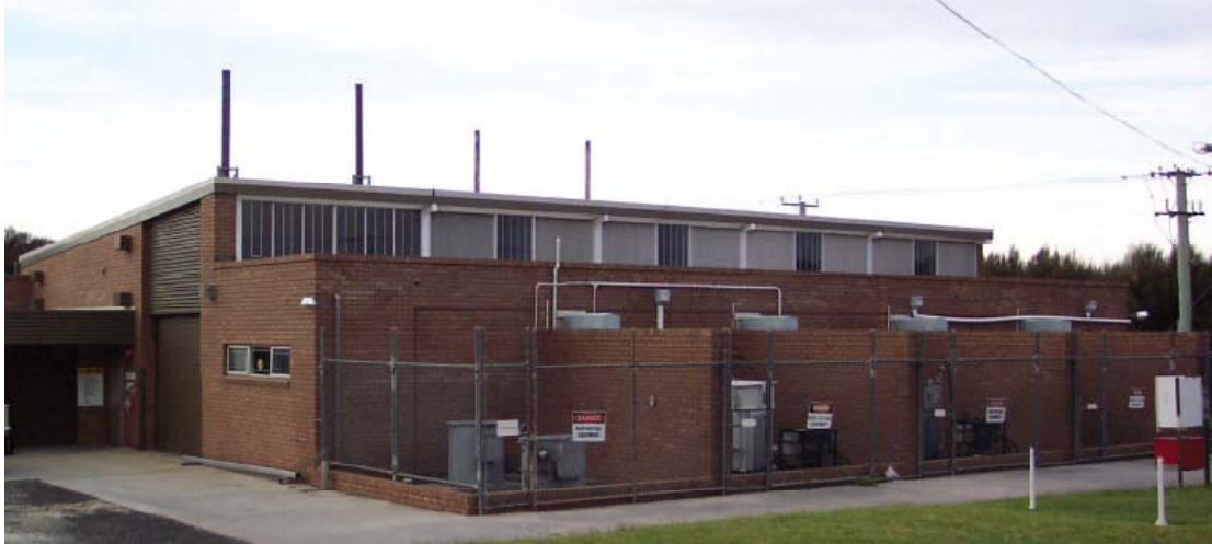
Figure 2.1: Whitemark Power Station, Flinders Island
